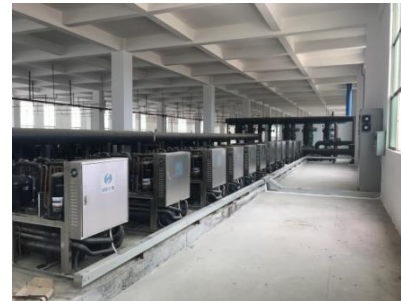
Large-scale green air-conditioning system
